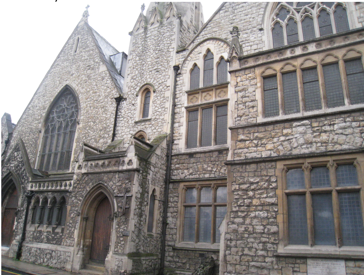
FRONT ELEVATION (145C TO THE LEFT (NOT PART OF APPLICATION) AND 145H TO THE RIGHT)
