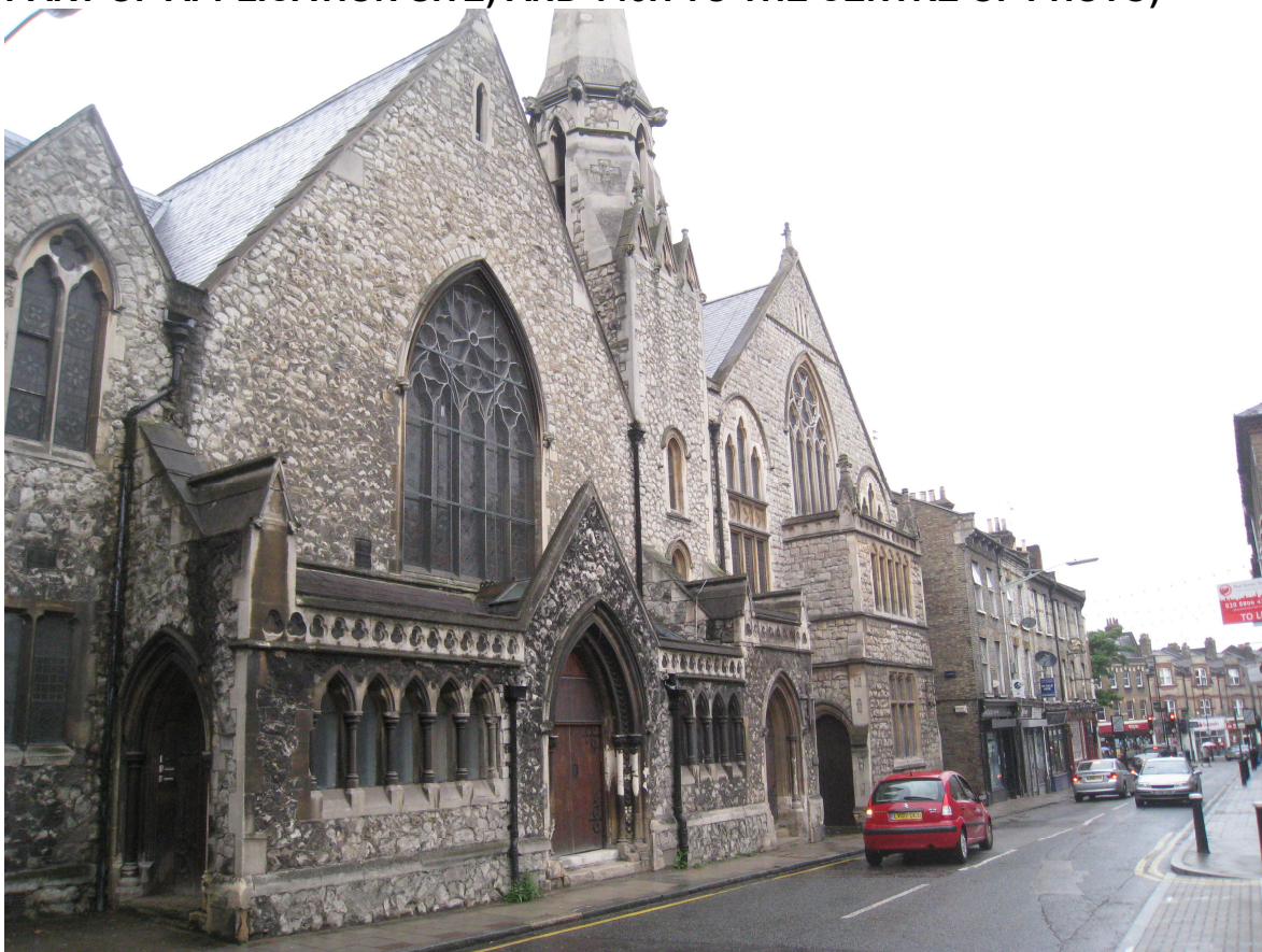
VIEW NORTH TOWARDS CROUCH END TOWN CENTRE (145C TO THE LEFT (NOT PART OF APPLICATION SITE) AND 145H TO THE CENTRE OF PHOTO)
